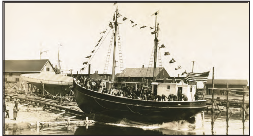
The Muskegon launches at I.L. Snow & Company in 1937 in Rockland. The 72-foot by 18-foot all-wood scalloper and dragger had a 140-hp diesel engine but also main and mizzen sail.
